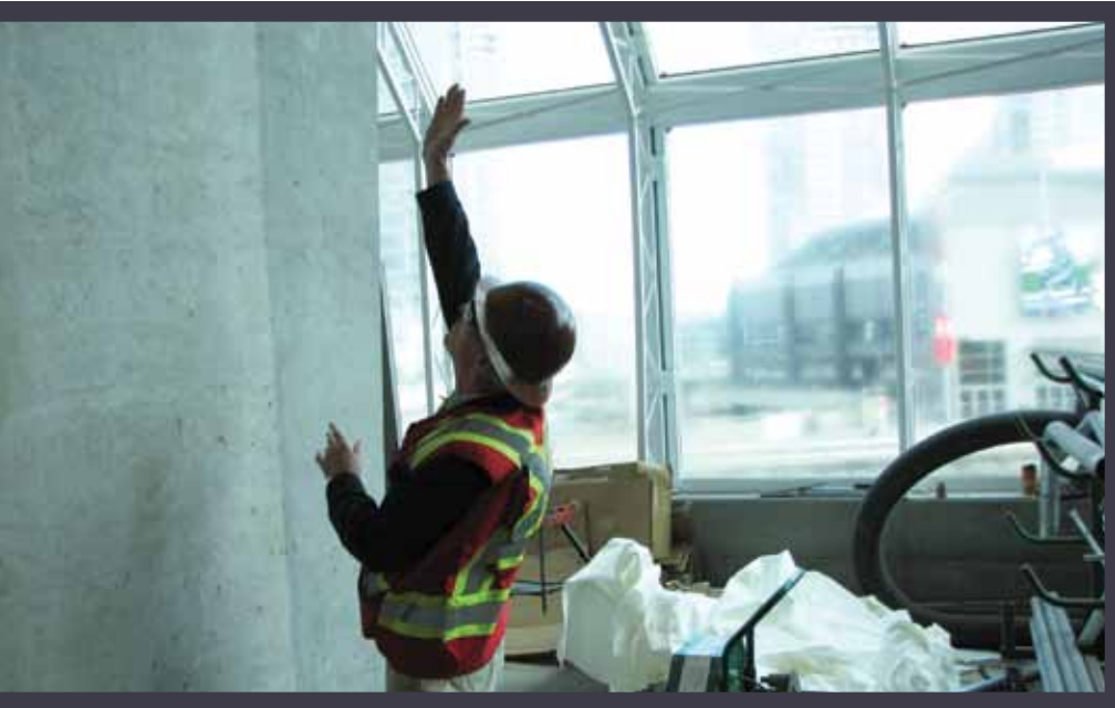
▲ PHOTO: MANY CHANGES AND IMPROVEMENTS HAVE GONE INTO THE ENTIRE FACILITY - NOT JUST THE ROOF.
